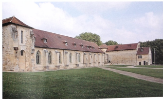
11 Abbey of Maubuisson, showing the conventual buildings from the east.
