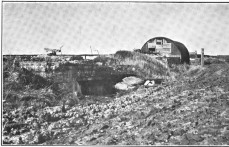
(B)—Remains of Concrete Blockhouse near Frezenberg—possibly the scene of Father Doyle's death. The shed on the right is a subsequent structure. (Photo taken at the position marked B on the Map on p. 540.)
