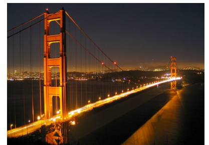
v / The Golden Gate Bridge's roadway is held up by the tension in the vertical cables.
