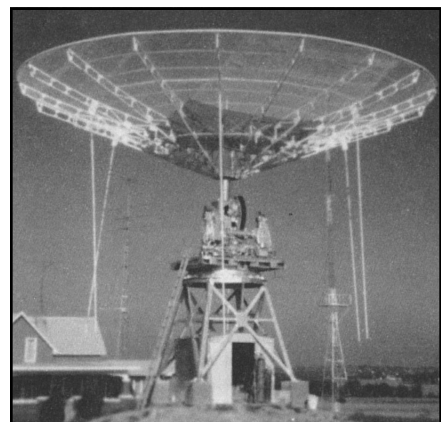
Fig 2—The gun mount of Fig 1 with its “warhead” attached—a home-made 42-foot parabolic dish. This is part of the arsenal of Ken Kucera, KAØY.
