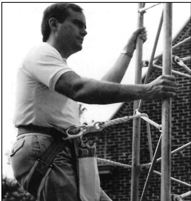
Fig 7—Mark Wilson, AA2Z, shows the proper way to attach a safety hook, with the opening facing away from the tower. That way the hook can't be accidentally released by pressing it against a tower leg.
