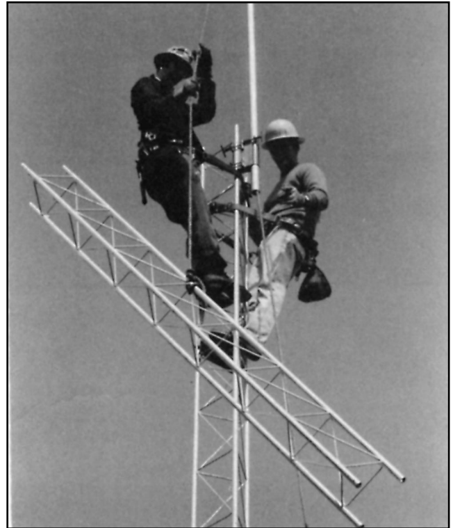
Fig 5—The assembly of tower sections is made simple when a gin pole is used to lift each one into position. Note that the safety belts of both climbers are fastened below the pole, thereby preventing the strap from slipping over the top section. (photo by K1WA)
