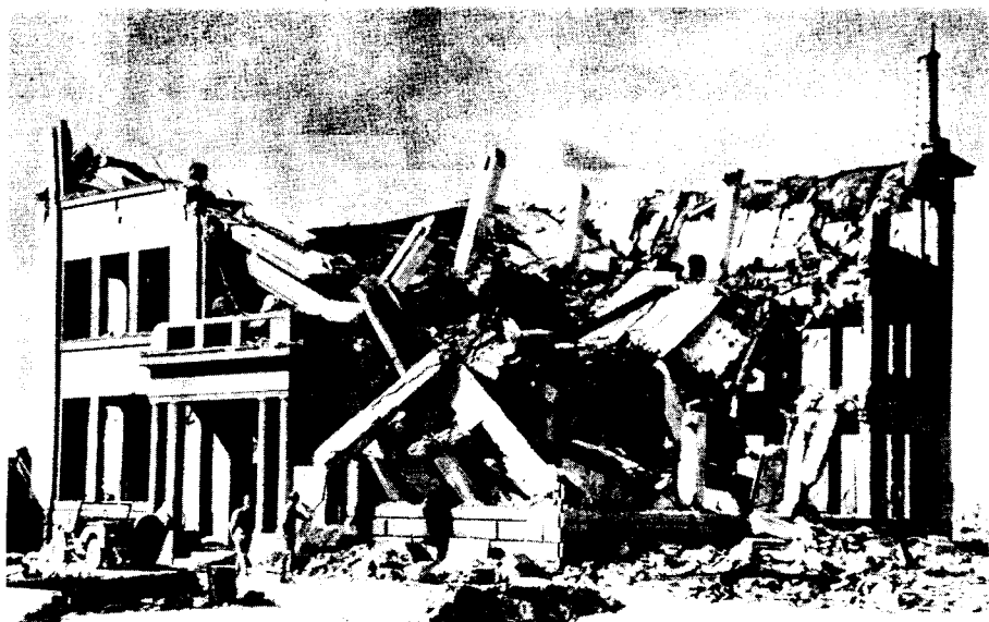
Figure 5.20b. Three-story, reinforced-concrete frame building; walls were 13-inch thick brick panel with large window openings (0.13 mile from ground zero at Hiroshima).
