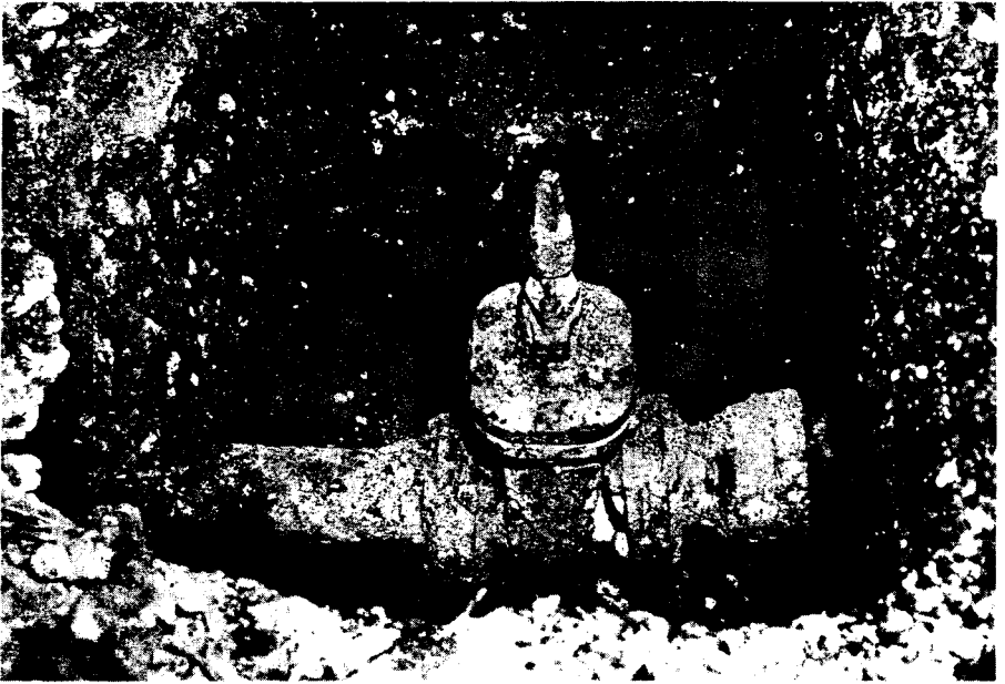
Figure 5.106a. Four-inch gate valve in water main broken by debris from brick wall (0.23 mile from ground zero at Hiroshima).
