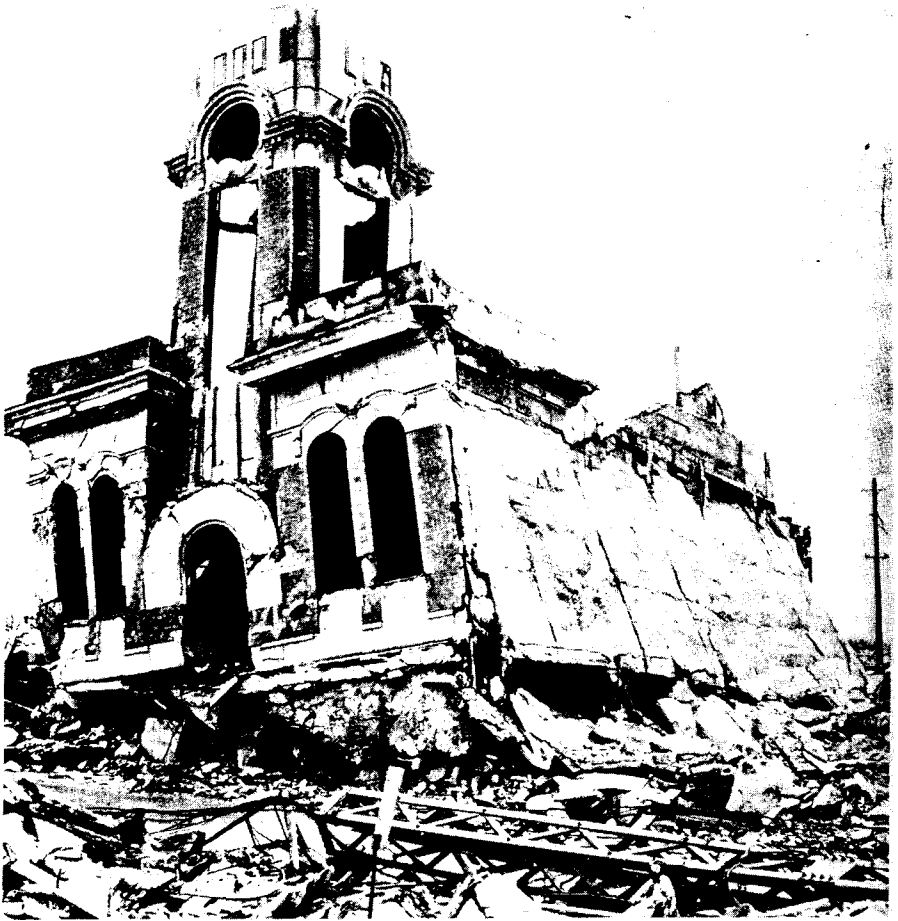
Figure 5.26. Two-story, steel-frame building with 7-inch reinforced-concrete wall panels (0.40 mile from ground zero at Hiroshima). The first story columns buckled away from ground zero dropping the second story to the ground.
