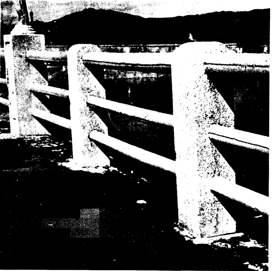
Figure 7.45a. Flash marks produced by thermal radiation on asphalt of bridge in Hiroshima. Where the railings served as a protection from the radiation, there were no marks; the length and direction of the "shadows" indicate the point of the bomb explosion.
