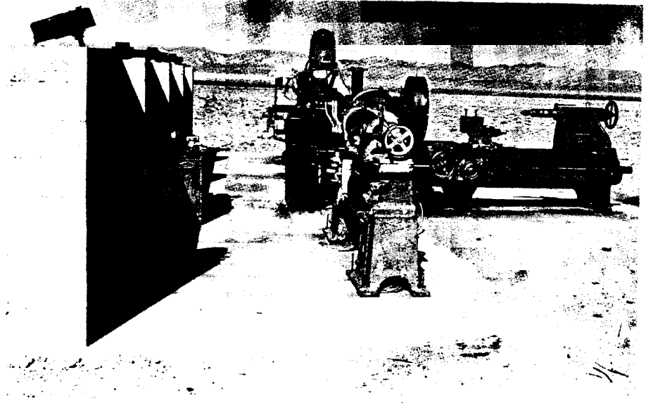
Figure 5.128. Machine tools behind masonry wall before a nuclear explosion, Nevada Test Site.
