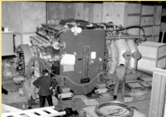
Installing the Heavy Liquid Bubble Chamber.
