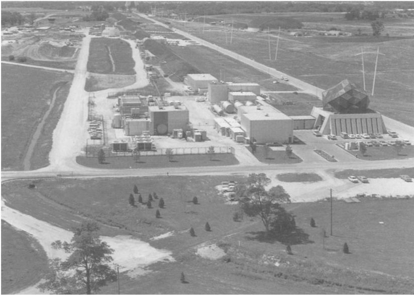
Fig. 19.4. The 15 foot bubble chamber sits at the end of the Neutrino Area. Adjacent is the Bubble Chamber Building, which is covered with a geodesic dome roof.
