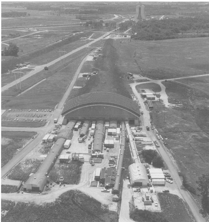
Fig. 19.3. The Meson Area, with its laboratory's distinctive roof, contains six particle beam lines.
