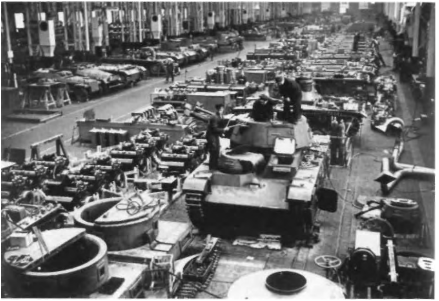
22. Rallying the home front with armaments propaganda: 'mass-production' of tanks as shown in German newsreels, May 1942.
