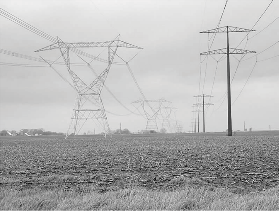
Figure 6-1. Transmission line right-of-way with two tower lines: single circuit lattice (left) and double-circuit tubular (right).
