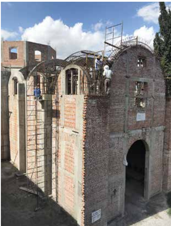
By August, 2019, work on the vaults began.
