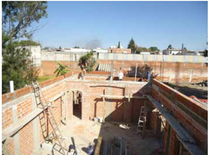
In January of 2016, the new presbytery rises from the ground.
