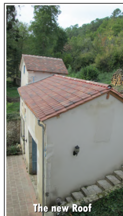
Repairing of the Roof of the Future Infirmary
